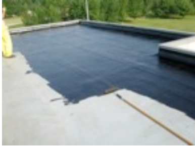
#229 Elastomeric “Brush” Applied over Primer on North Side Flat Roof (3 weeks dry time)
