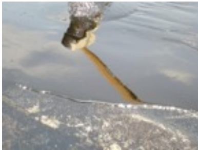
#229 Elastomeric “Brush” Applied over Primer on North Side Flat Roof (3 weeks dry time)
