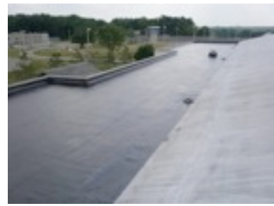
#229 Elastomeric “Brush” Applied over Primer on North Side Flat Roof (3 weeks dry time)
