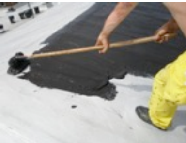
#220 Asphalt Emulsion Fibered applied to Sloped roof areas (3 weeks Dry Time)
