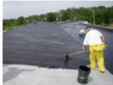
#220 Asphalt Emulsion Fibered applied to Sloped roof areas (3 weeks Dry Time)
