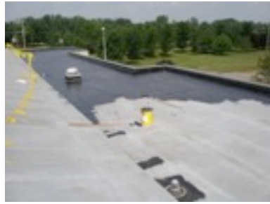
#229 Elastomeric “Brush” Applied over Primer on North Side Flat Roof (3 weeks dry time)
