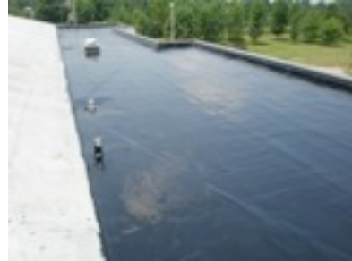
#229 Elastomeric “Brush” Applied over Primer on North Side Flat Roof (3 weeks dry time)
