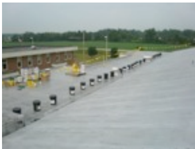
#220 Asphalt Emulsion Fibered applied to Sloped roof areas (3 weeks Dry Time)
