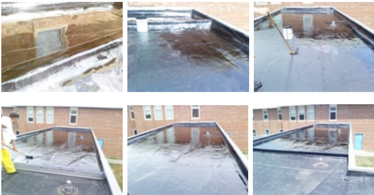
#229 Elastomeric “Brush” Applied over Primer on Breese Way Flat Roof (3 weeks dry time)
