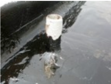
#229 Elastomeric “Brush” Applied over Primer on North Side Flat Roof (3 weeks dry time)
